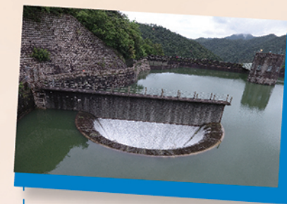
鐘形溢流口 Bellmouth Overflow
