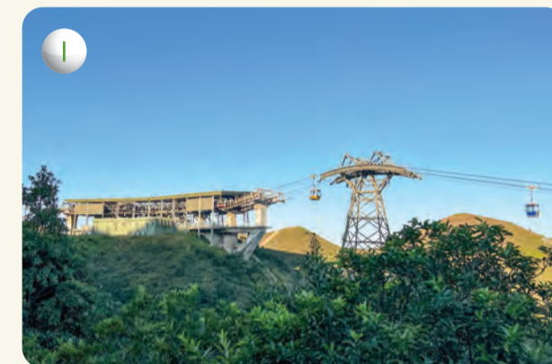
彌勒山轉向站 Nei Lak Shan Angle Station
