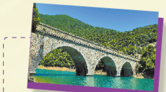
大潭水塘 Tai Tam Reservoir
